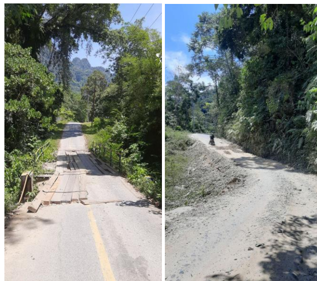
Figure 3. current condition of road access to Silokek Geopark
