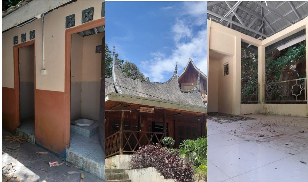
Figure 1. Current Condition of Facilities At Geopark Silokek Area
