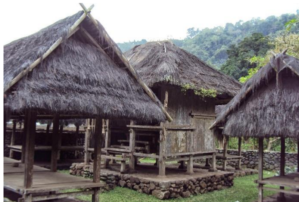
Figure 3. Use of natural materials on roofs, poles, walls, and floors in buildings in Tenganan village Source: Commons Wikimedia, 2009
