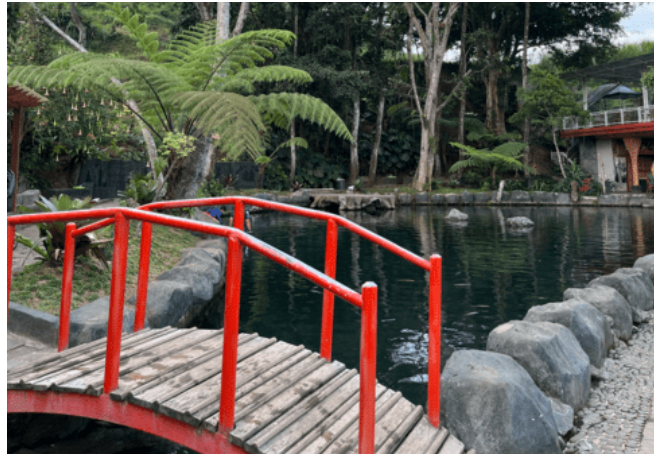
(Side view of Telaga Madiredo with the newly built bridge)
